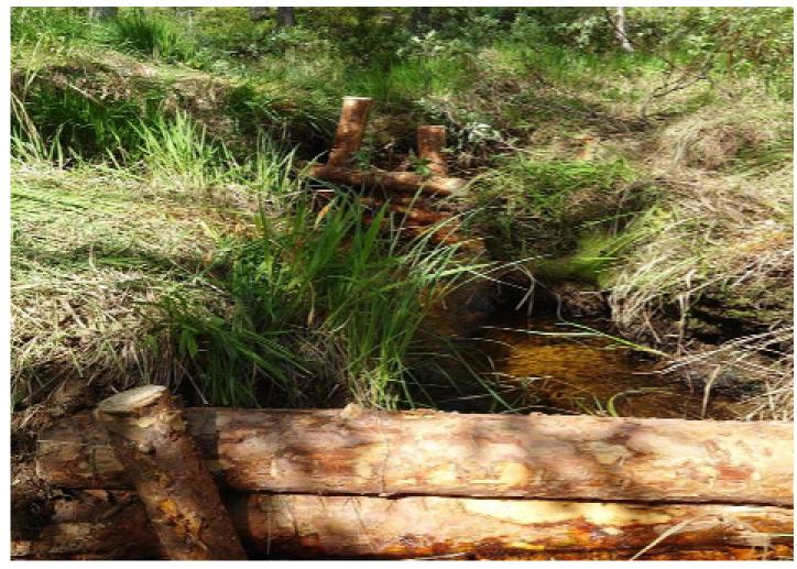
Timber structures (deflectors) that stop the flow of water and even out the water speed. Small streams like this obtain some dead wood in them and this provides more oxygen, food for insects and helps to remove fine particles from the stream.
